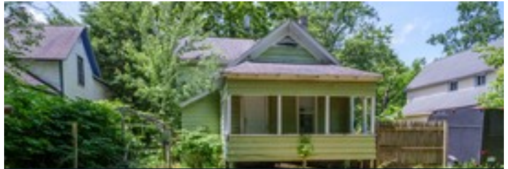
1135 March Street 3-Unit Multifamily
