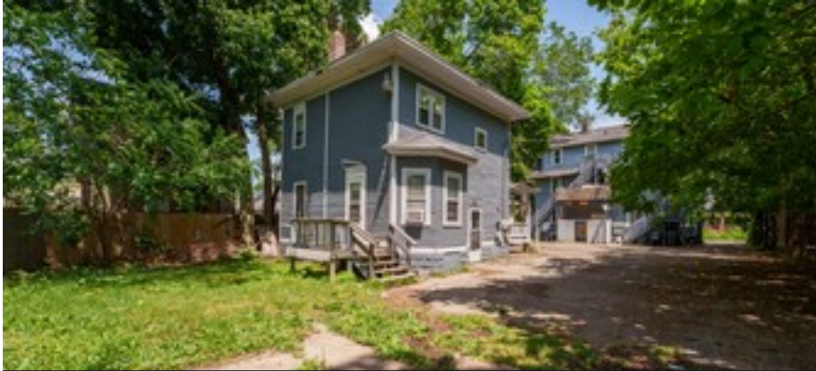
906 & 908 S Park Street 6-Unit Multifamily | Kalamazoo, MI
