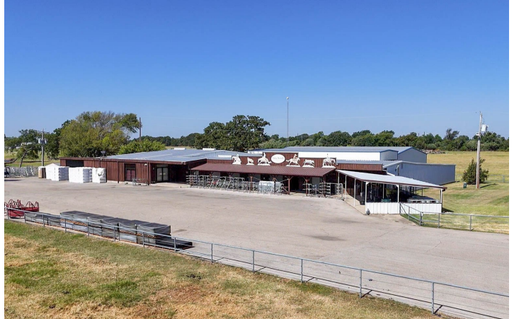
Main Warehouse / 100% HVAC
