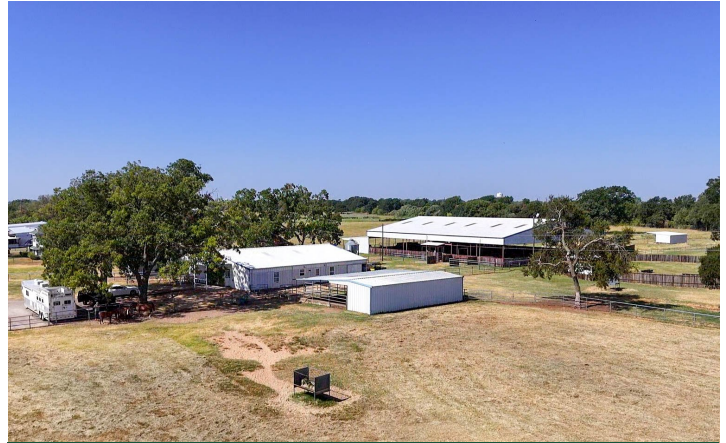
Covered Arena / Barns
