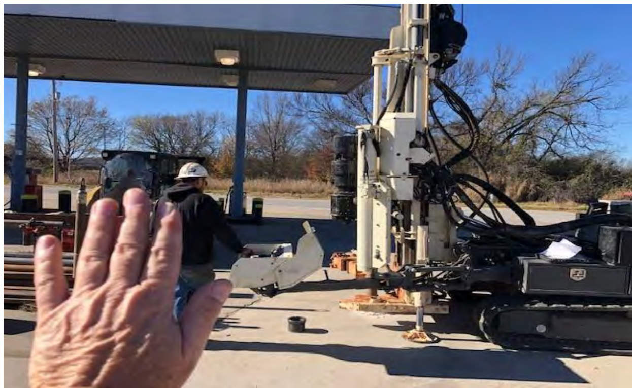
SOIL BORING SB-5 LOCATION
