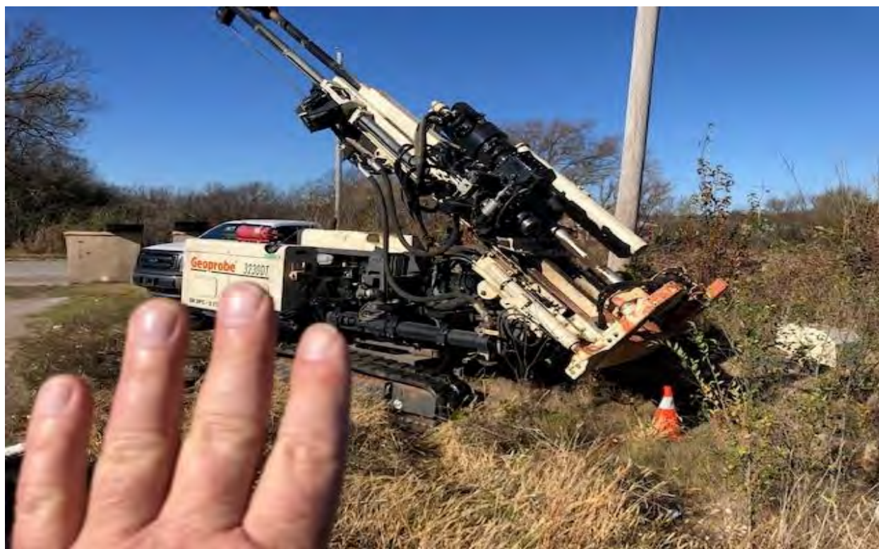
SOIL BORING SB-4 LOCATION
