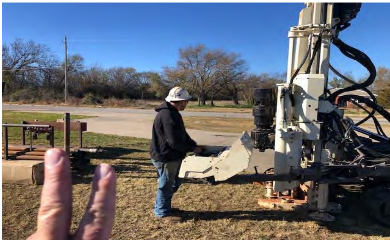
SOIL BORING SB-2 LOCATION
