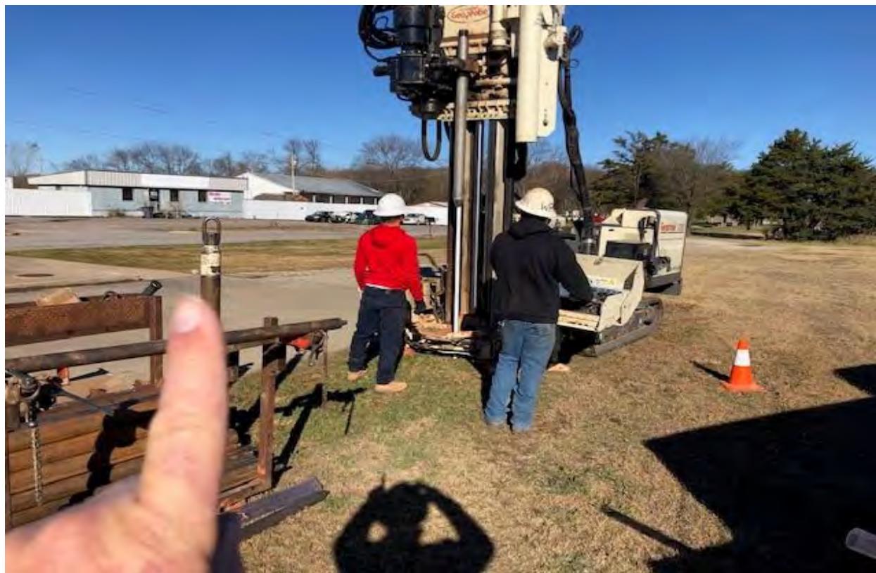
SOIL BORING SB-1 LOCATION
