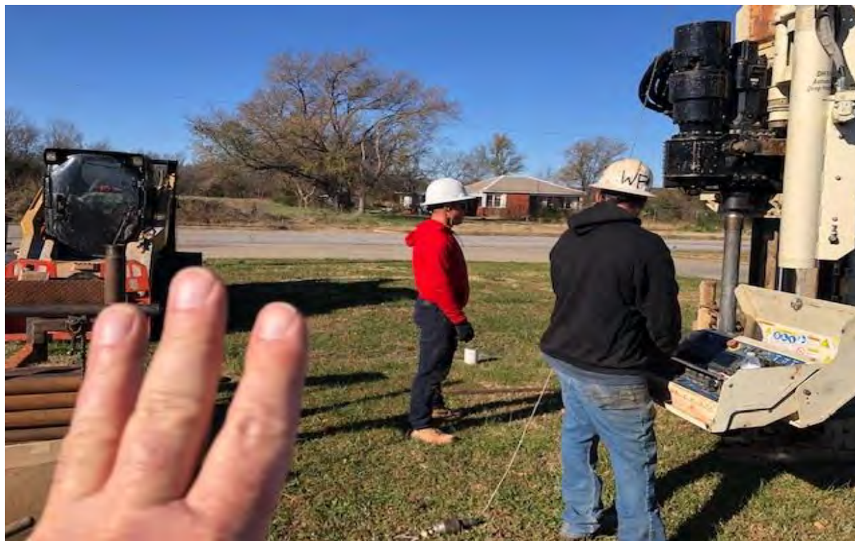
SOIL BORING SB-3 LOCATION
