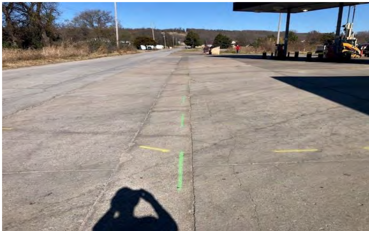
UTILITIES WEST SIDE FACILITY
