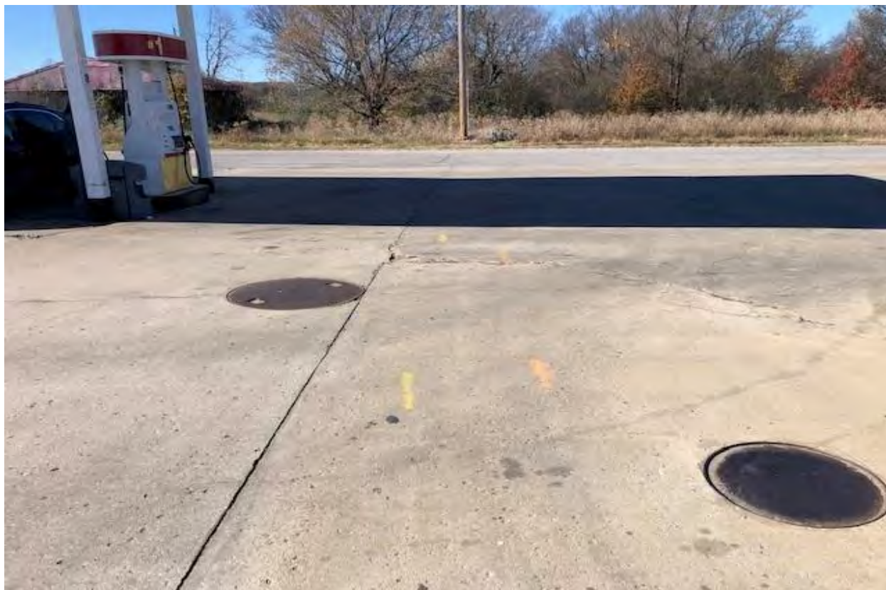
LINE SUMPS BETWEEN DIESEL AND GASOLINE DISPENSERS AND CANOPIES
