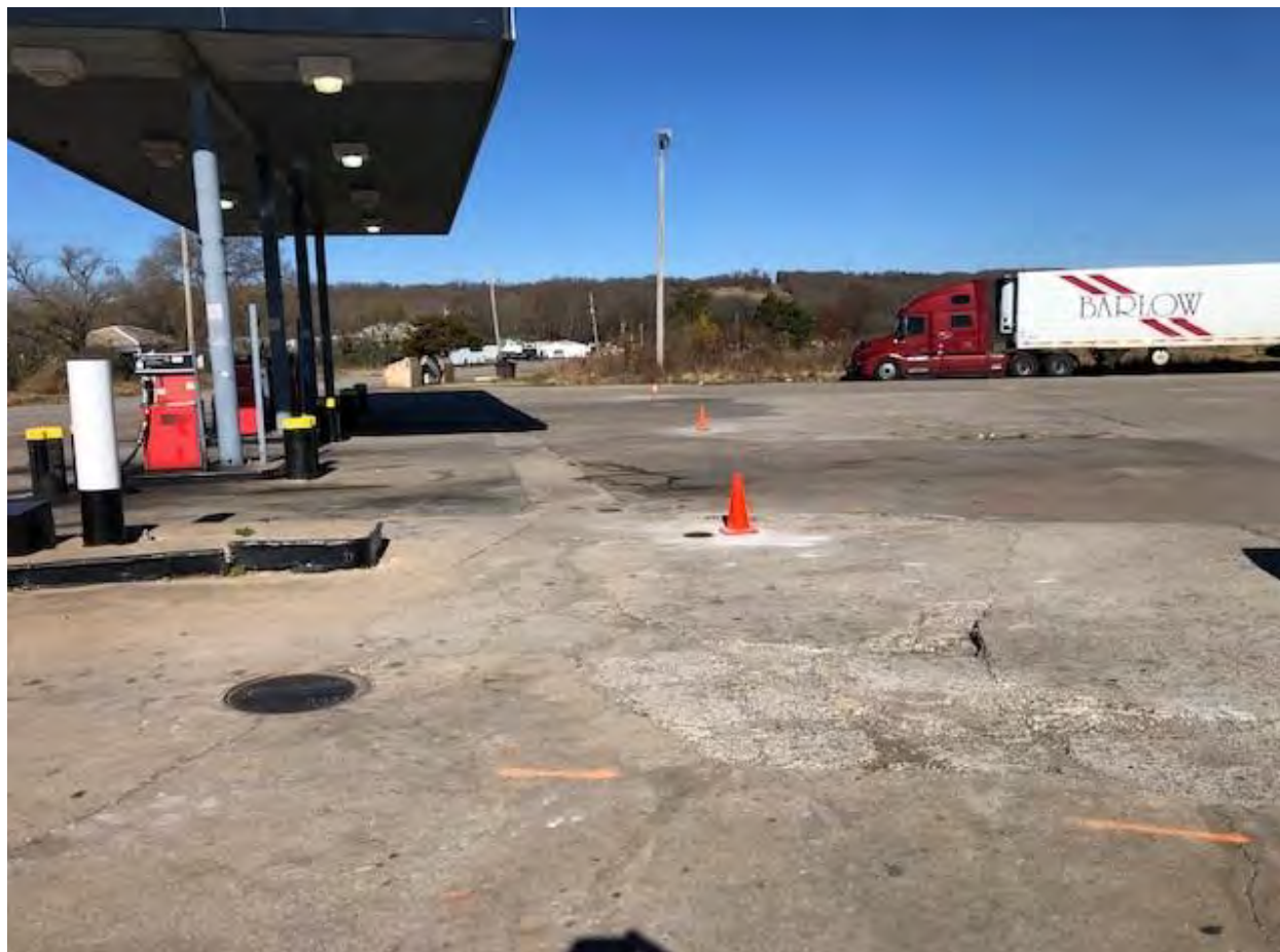
PLUGGED SOIL BORING SB-5, SB-6 AND SB-7
