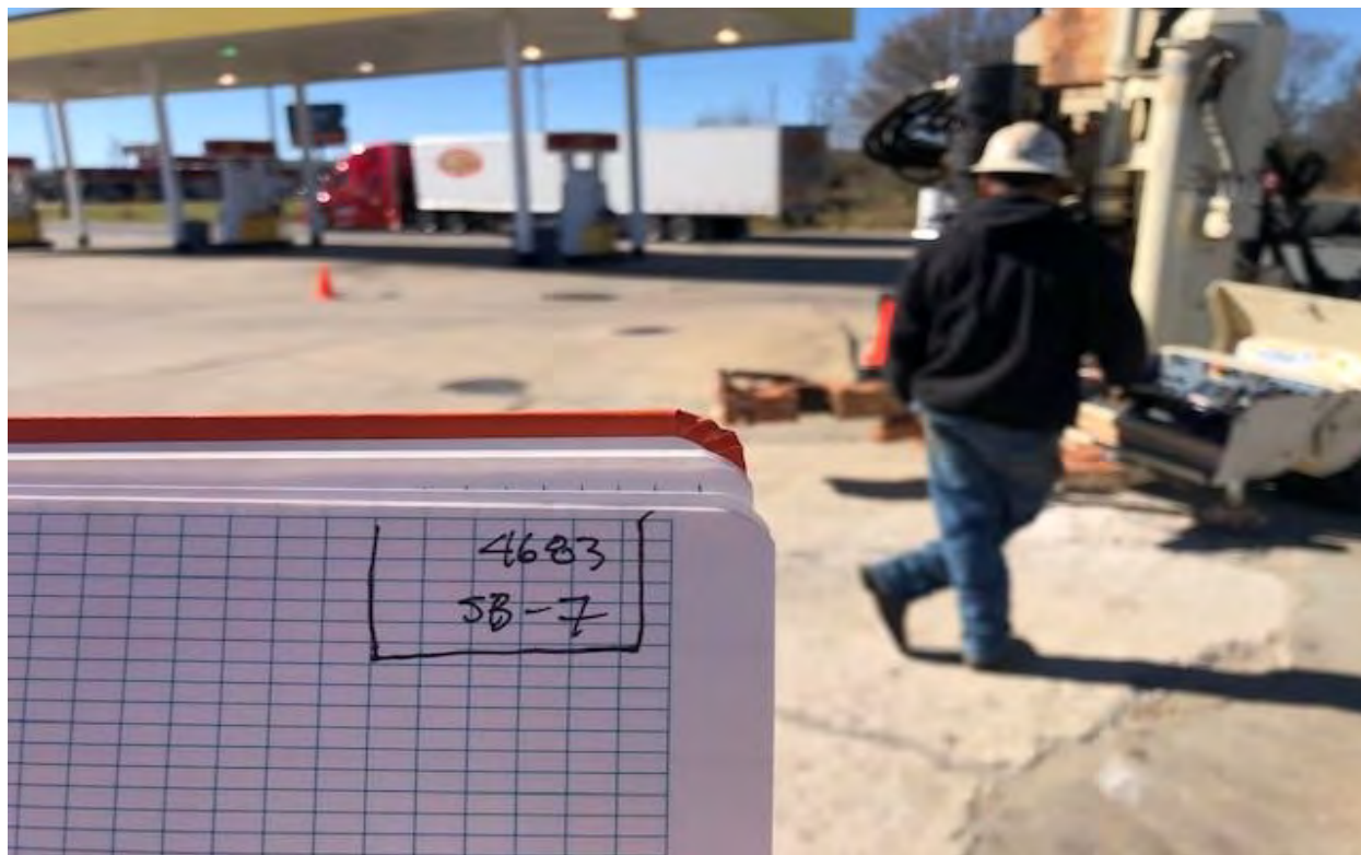
SOIL BORING SB-7 LOCATION
