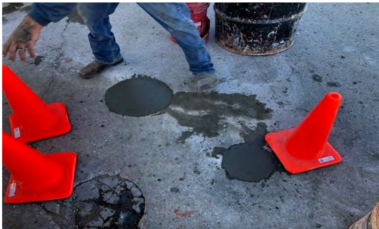
SOIL BORING SB-8 LOCATION, DRILLED AND PLUGGED, REPAIR OLD WELL SURFACE
