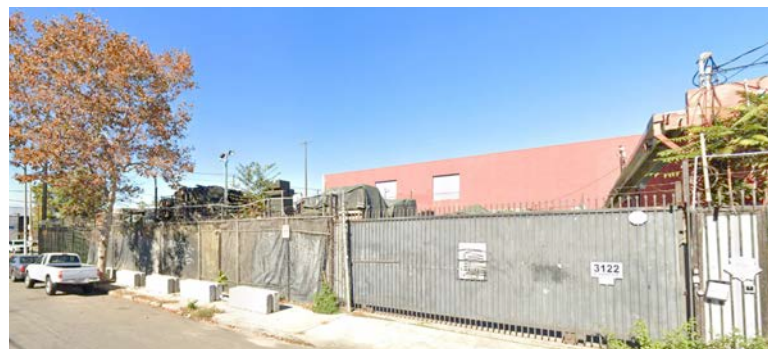
32nd Street access point adjacent to the building supporting internal circulation and operational flow
