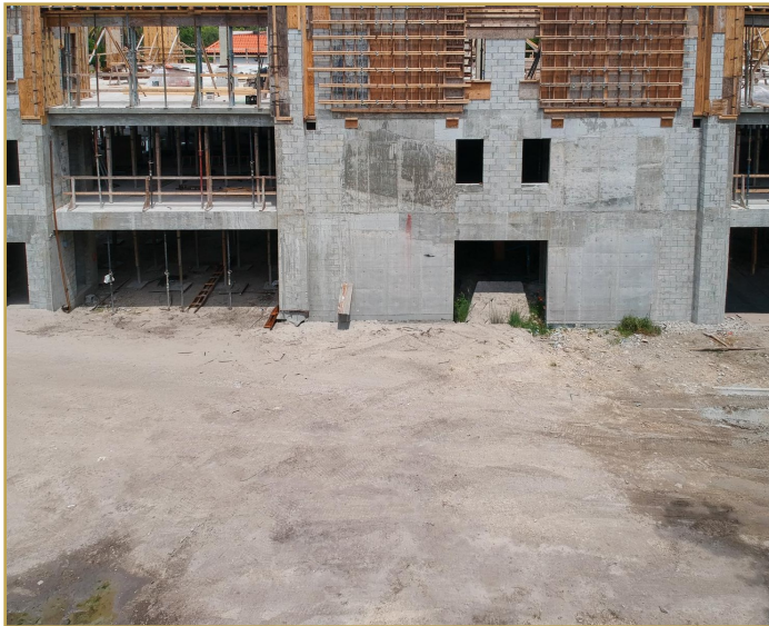
Exterior wall formwork in progress
