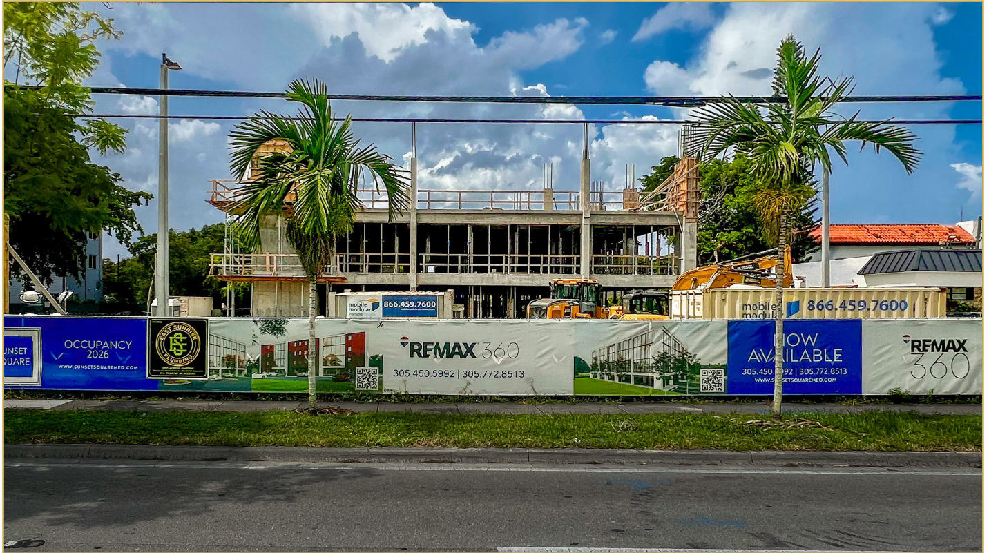
Sunset Square site frontage on Sunset Drive
