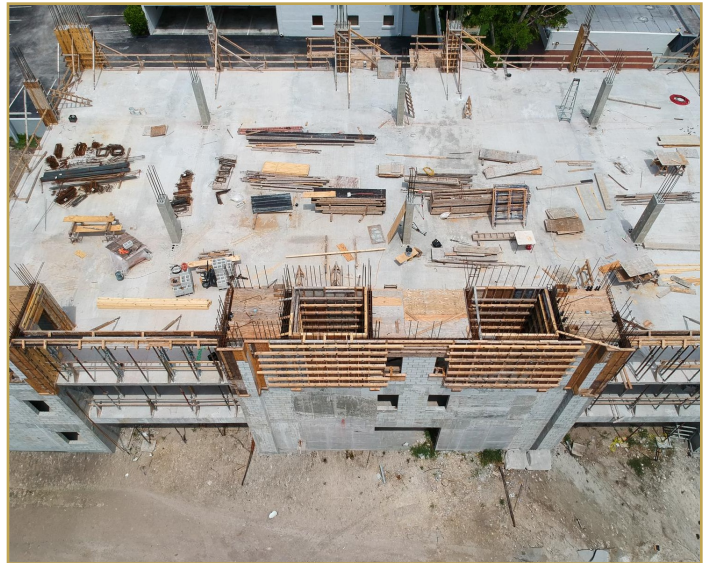
Aerial view of second-floor slab and framing
