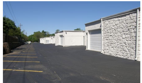
Back Section/OH Door Access
