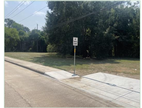
Curb, sidewalk and drive approach
