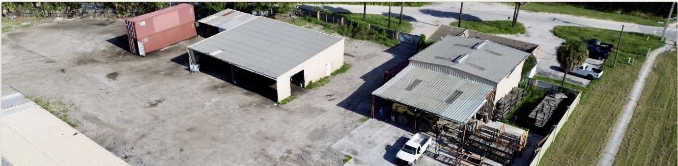
SITE OVERVIEW — FOUR STRUCTURES ON A FENCED, STABILIZED ±5-ACRE YARD
