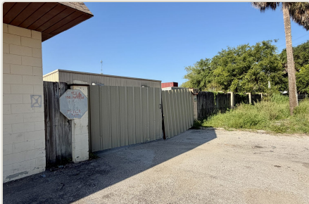
Gated, secured site access
