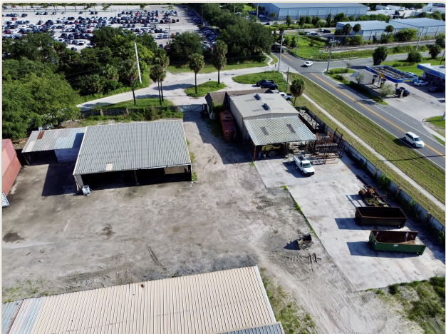
AERIAL LOOKING TOWARD ALBRIGHT RD — RAIL LINE, RETAIL FRONTAGE & AIRPORT PARKING BEYOND
