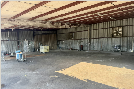
Clear-span warehouse interior
