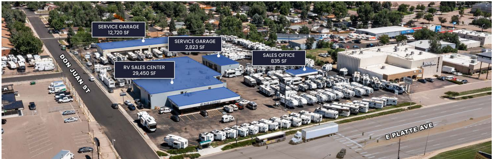
(1) New TPO roof over showroom in 2019. New TPO installed over sales center in 2024.
