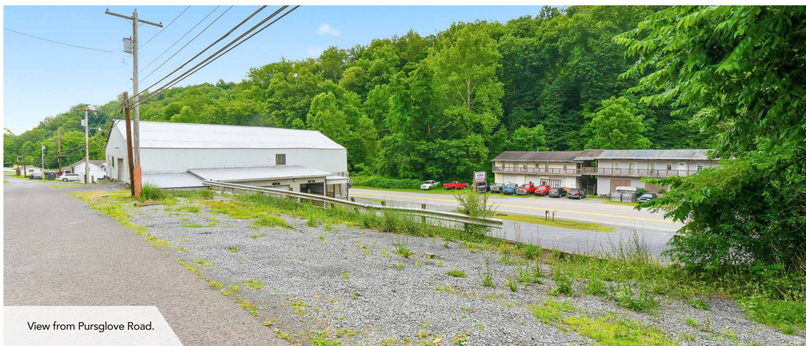
Upper Level Access.
