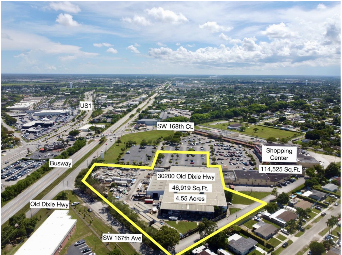
±4.5-acre site fronting Old Dixie Highway, one block off US-1 and the Busway, adjoining a 114,525 SF anchored shopping center.
