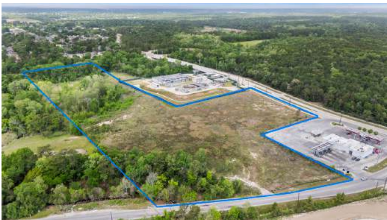
VIEW OF PROPERTY LOOKING NORTH
