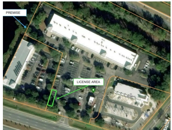
Electric Vehicle Charging stations 'coming soon'
