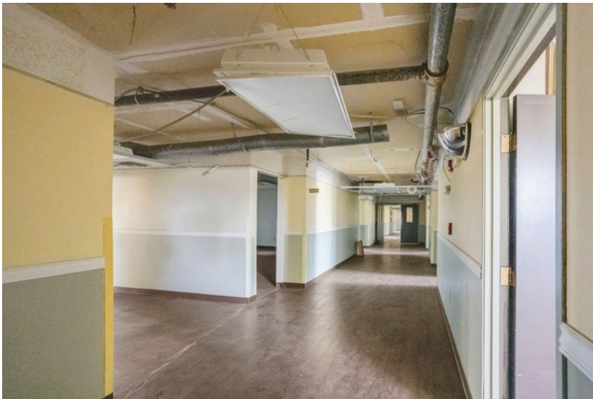
Representative unit interior in current shell condition following prior ownership demolition
