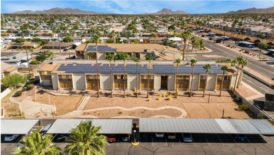
Aerial view: north elevation, parking, and rooftop solar array
