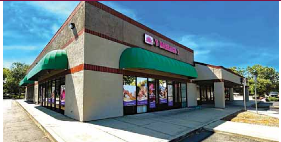
NEW EXTERIOR PAINT
