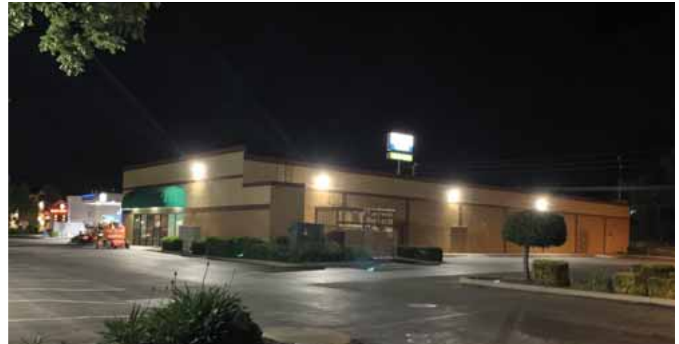
NEW LED OUTDOOR LIGHTING UPGRADED
