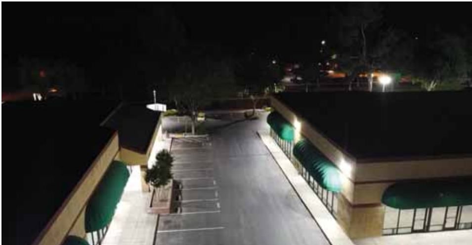
NEW LED OUTDOOR LIGHTING UPGRADED
