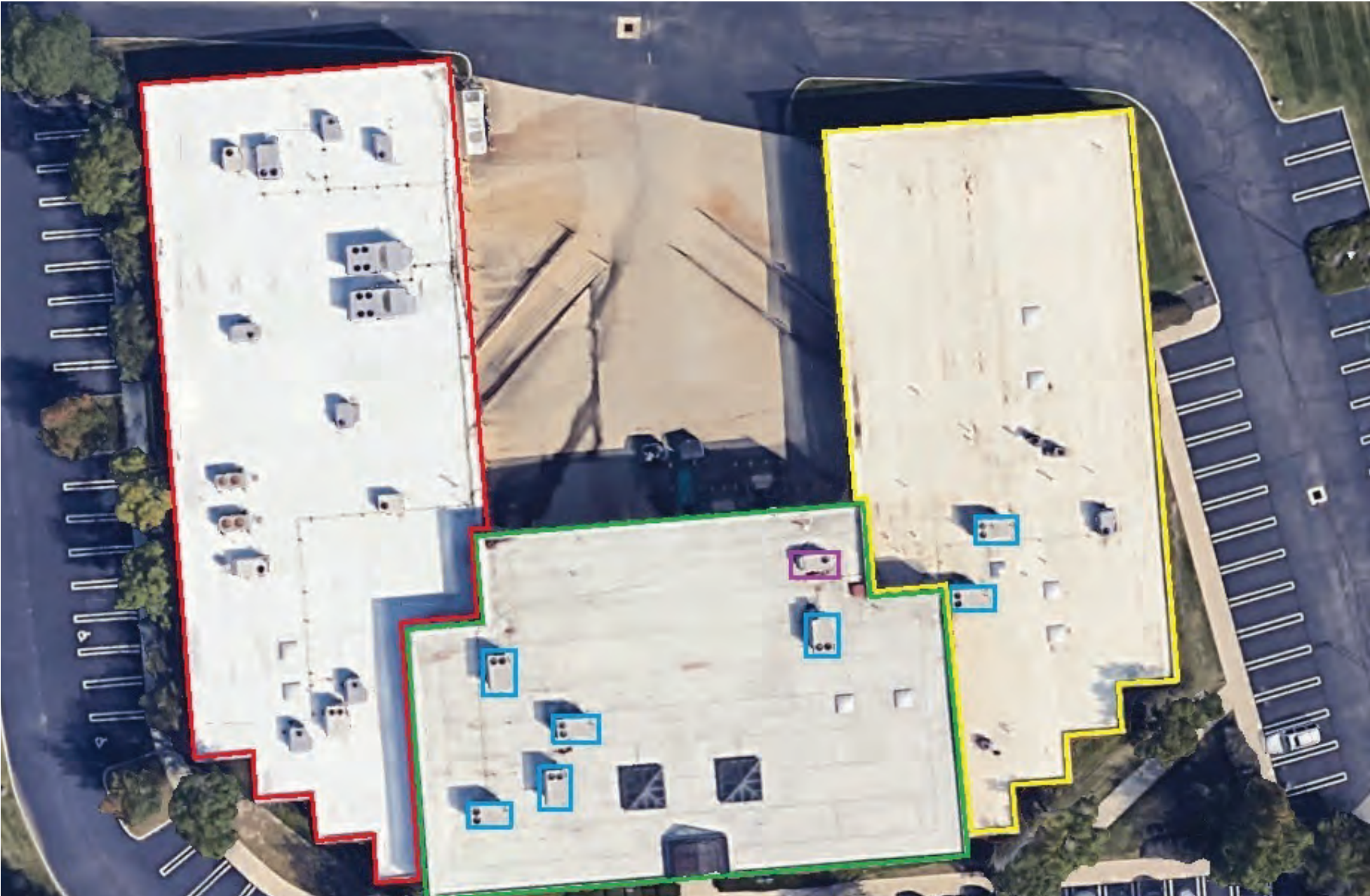
HVAC & Roof replacement/warranty information to follow on the next page.
