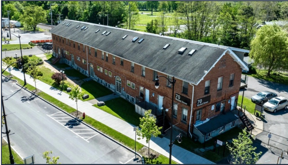
70 Market Street — 24-unit brick building
