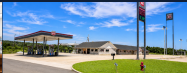
WIDE SITE VIEW
