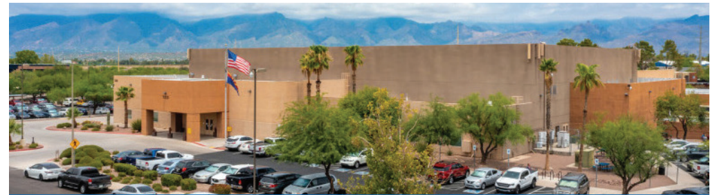
Western Passport Center | Tucson, AZ (±75,000 SF)
