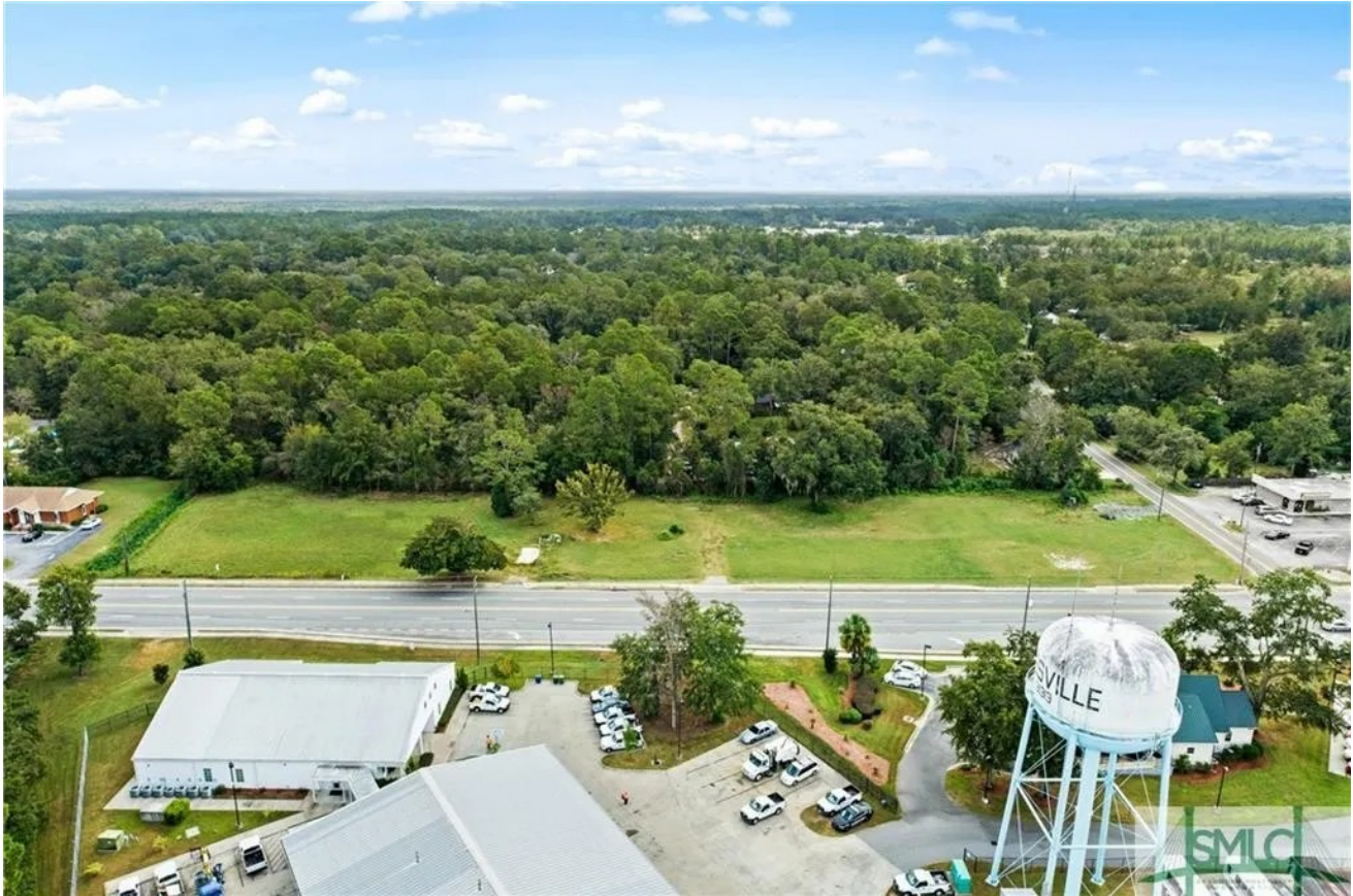
Existing corridor-facing property photograph supplied by ownership.
