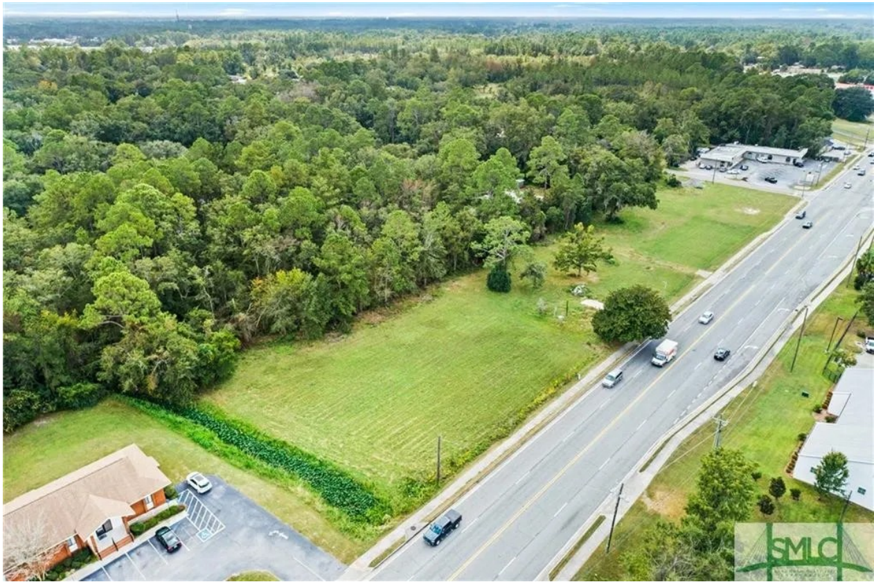
Ownership-supplied aerial view of the development site.
