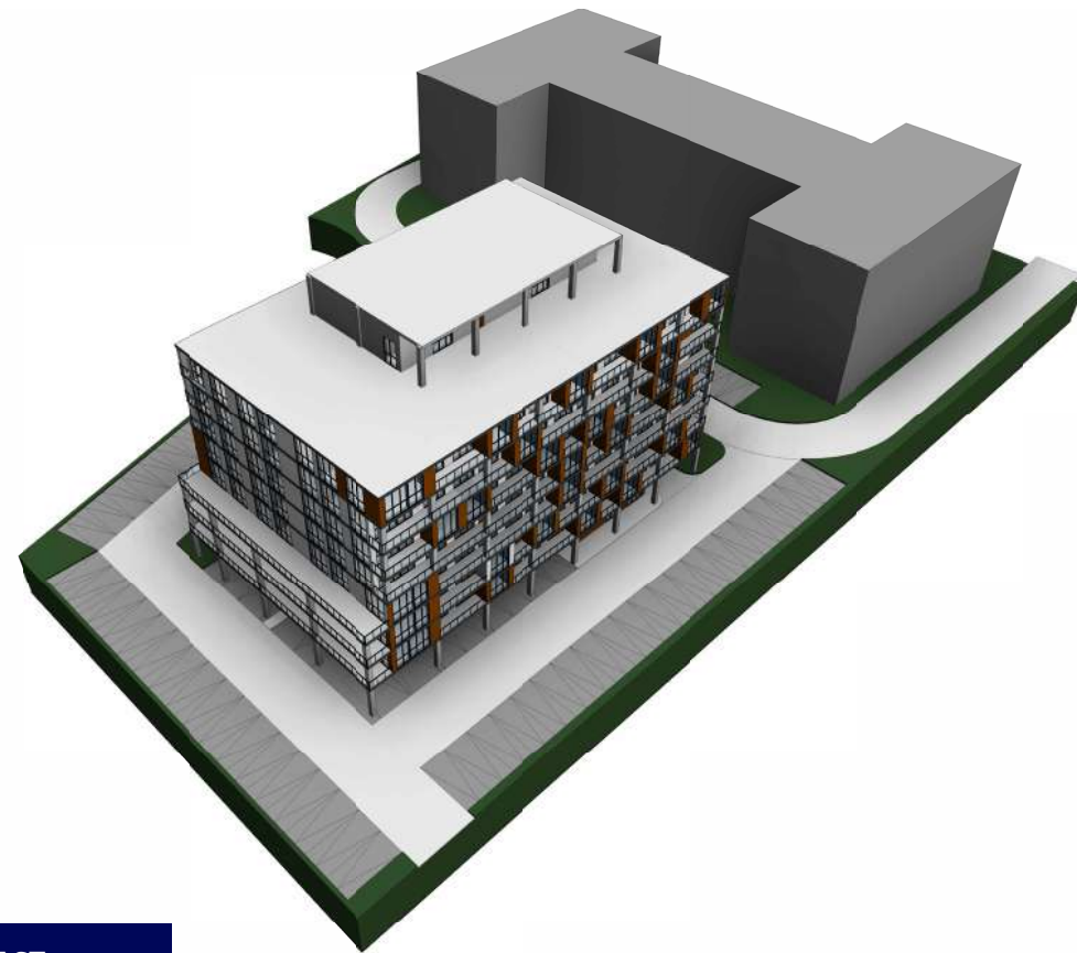
AERIAL LOOKING EAST
