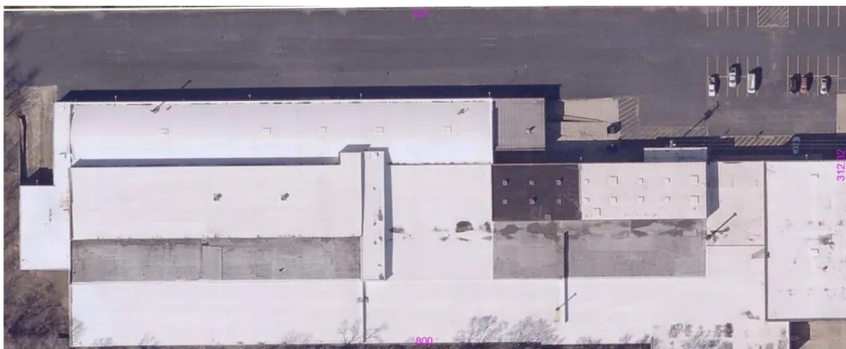
Aerial view showing individual roof sections. Full inspection report available in the diligence package.
