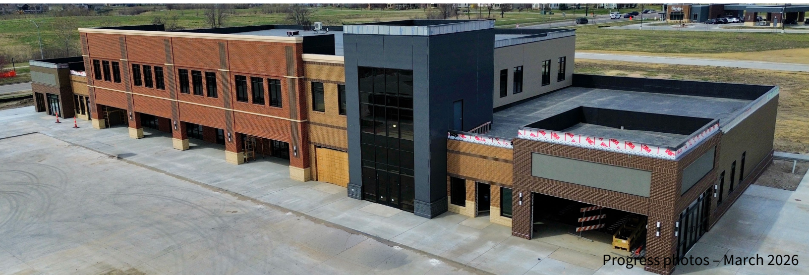
Progress photos – March 2026
