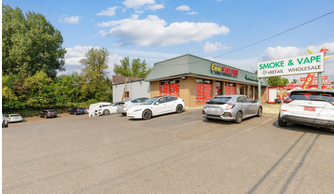
Front parking and access
