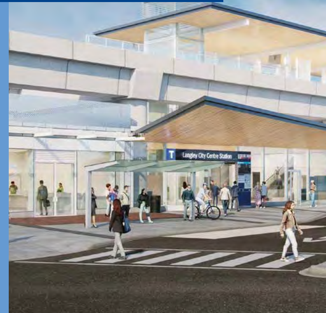
Langley City Centre Station
