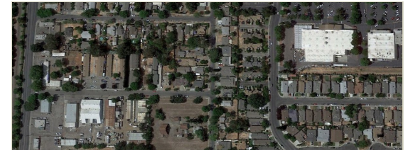
Aerial context — Johnston Street corridor, Downtown Woodland
