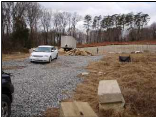
Stone-lined entrance drive, with storage trailer in background.
