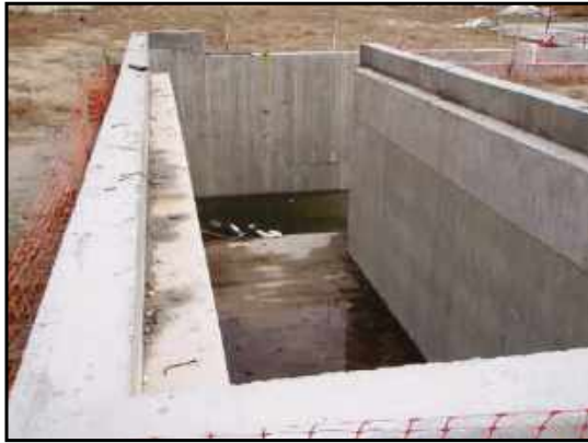
View inside concrete-lined pit on site.
