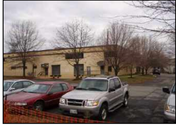
Alexandria Metal Finishers is located directly north of the subject property.
