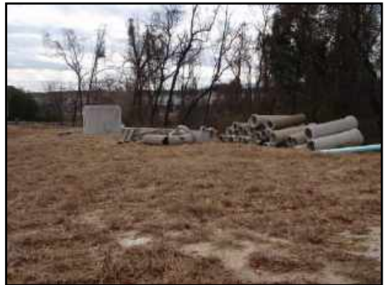
Precast concrete pipe and products on southern side of site.
