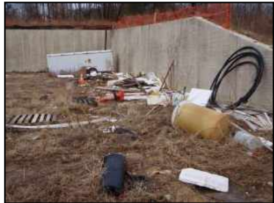
Miscellaneous trash and debris on northwest corner of site, with retaining wall in background. Note small storage trailer and 55-gallon drum.
