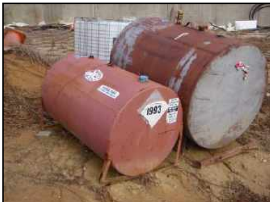
The two smaller aboveground tanks on the site, presumed to be 300-gallon and 100-gallon tanks. The smaller (100-gallon) tank was marked to contain off-road diesel fuel, and may contain a small amount of petroleum.
