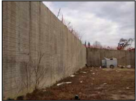
Retaining wall on western side of site.
