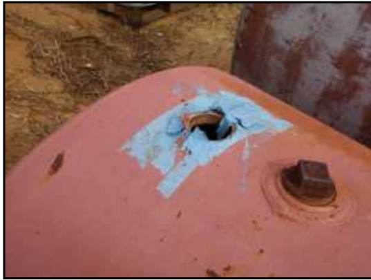
The lack of a tape cap on the smaller (100-gallon) aboveground tank may have let rainfall in; the tank appears to contain a small volume of liquid with a petroleum odor.
