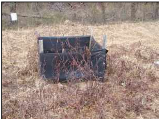
Silt fence around manhole that is part of on-site drainage system.
