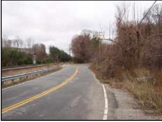
Gunston Cove Road in front of subject property, looking to south.
