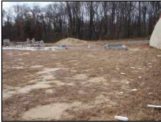
Concrete pad within interior of site.
