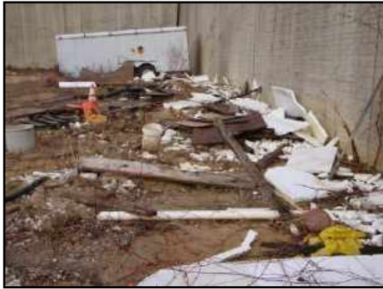
Debris at northwest corner of site. Note small storage trailer.
