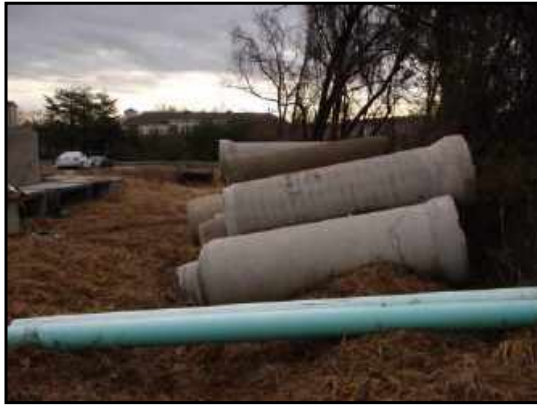
Precast concrete pipes and plastic pipes on subject property. These may have been used in connection with site construction.
