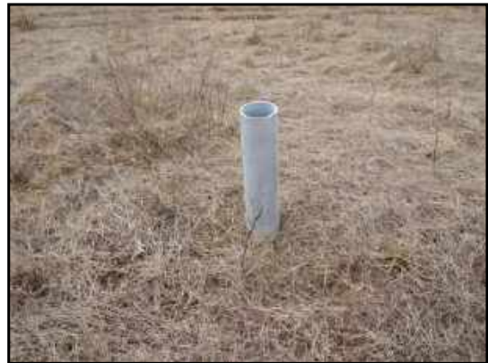
A standpipe is present on the site, which appears to contain features associated with the drainage or water system of the site due to its location (it was filled with water during the inspection).
