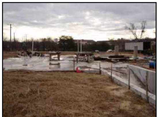
Concrete pad under construction at subject property.
