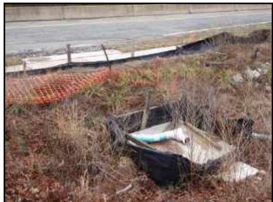
Manhole associated with on-site drainage system at northeast corner of site.
