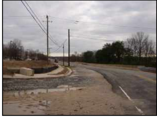
Gunston Cove Road in front of subject property, looking to north. The subject property includes a paved sidewalk along the roadway.
