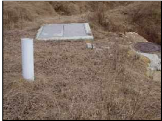
Structures associated with on-site drainage system.
