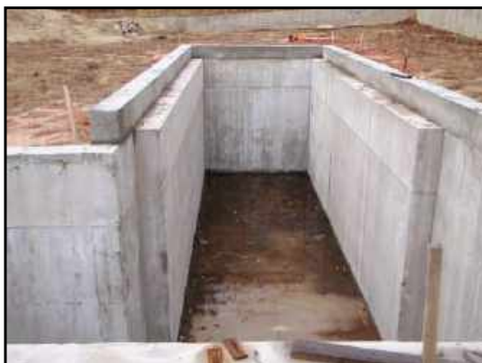
View inside concrete-lined pit.
