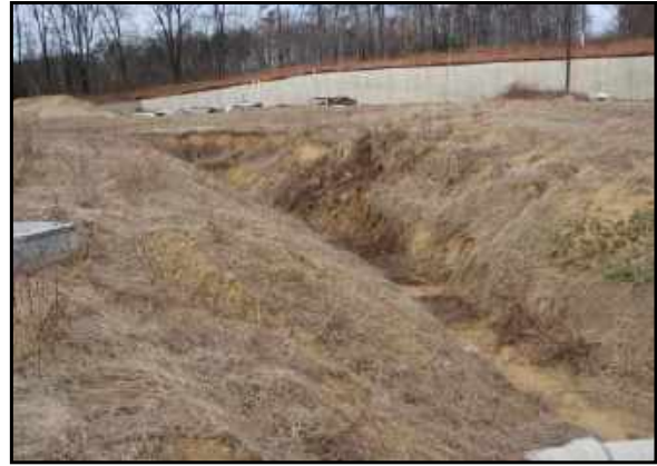
Drainage gully on site, which may have been excavated, looking to west side of site.
