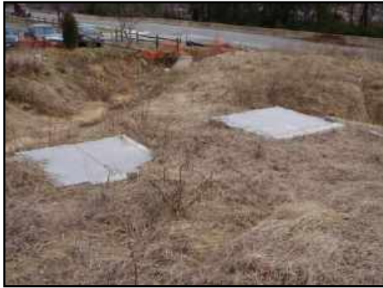
Structure associated with on-site drainage system.
