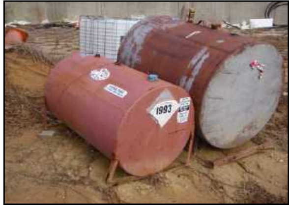
The two smaller aboveground tanks on the site, presumed to be 300-gallon and 100-gallon tanks. The smaller (100-gallon) tank was marked to contain off-road diesel fuel, and may contain a small amount of petroleum.
