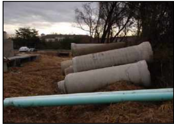
Precast concrete pipes and plastic pipes on subject property. These may have been used in connection with site construction.
