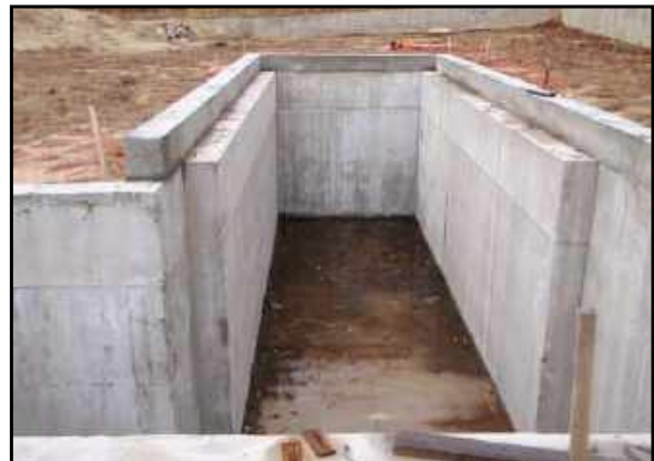
View inside concrete-lined pit.
