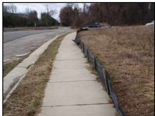
Concrete sidewalk in front of subject property along Gunston Cove Road, looking to south.
