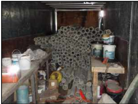
Materials stored inside storage trailer.
