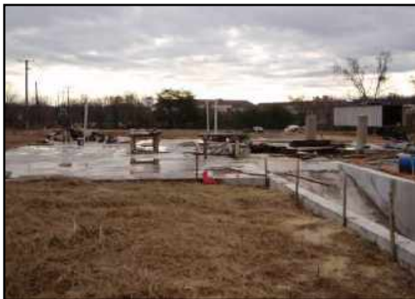
Concrete pad under construction at subject property.
