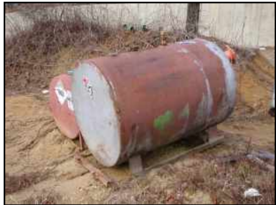
Two smaller aboveground storage tanks on subject property, located in the center of the site. Shown is a 300-gallon tank and a smaller 100-gallon tank (both sizes assumed, tanks not marked to size). Both tanks appear empty (the small tank may contain a small volume of petroleum), and no spills, leaks or stained soils
