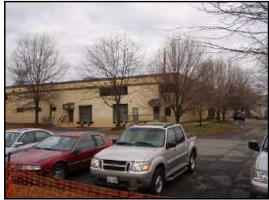
Alexandria Metal Finishers is located directly north of the subject property.
