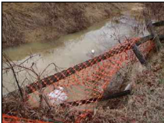
Water ponded within gully at northeast corner of site.
