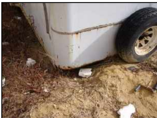
Bottom of small storage trailer. No staining of the ground around the perimeter of the trailer was observed.
