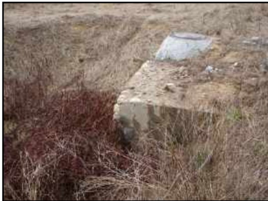
Concrete pad around manhole associated with on-site drainage system.
