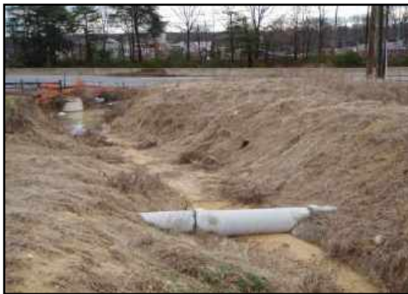
Gully on subject property, looking towards northeast corner of site. Drainage pipe is visible crossing the gully, which appears to be part of the on-site drainage system.
