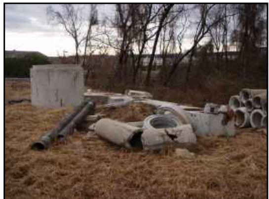
Precast concrete pipes, vault, and other materials on southern side of site.
