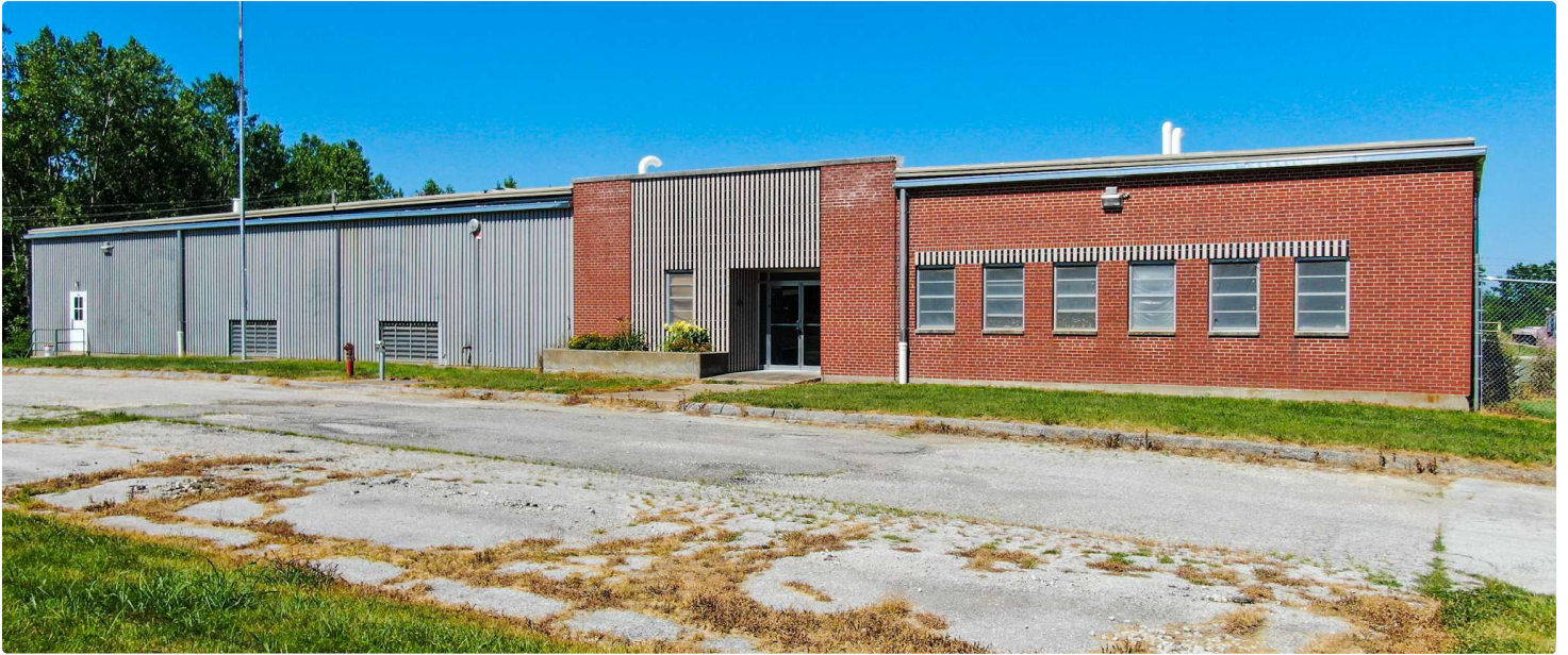
Front elevation, brick office frontage with primary entrance
