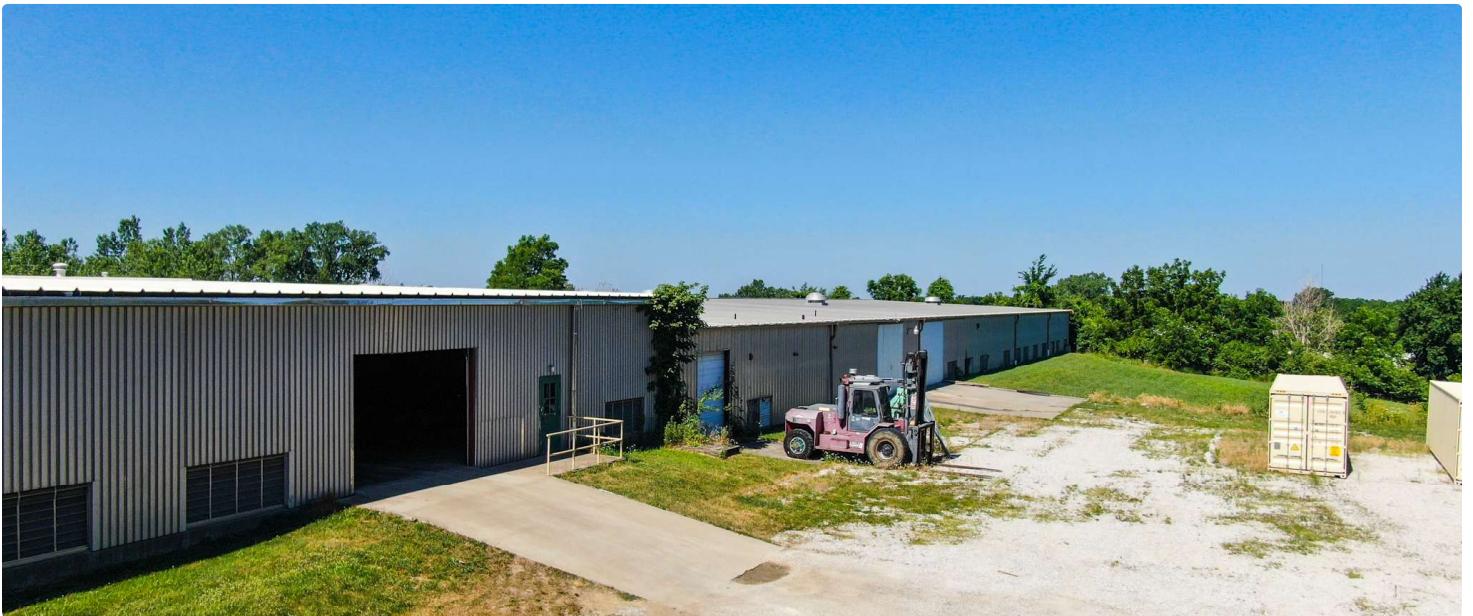
Drive-in and dock-high loading access serving the warehouse
