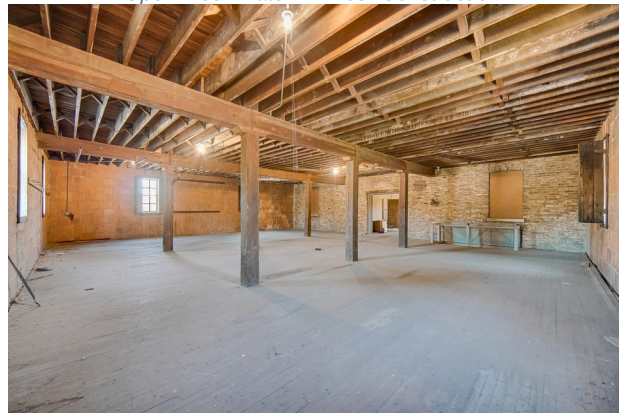
Open Floor Plate – Heavy Timber Framing
