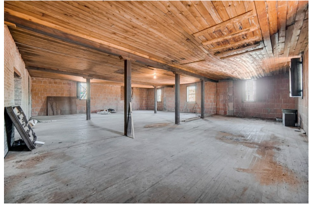
Open Floor Plate – Timber Construction
