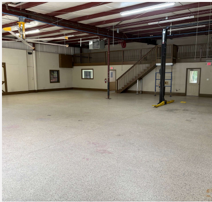
Warehouse bay with mezzanine above
