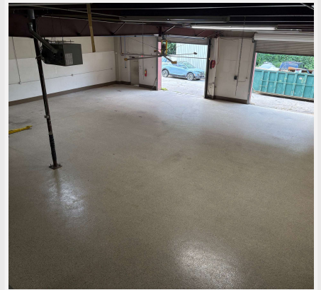
Grade-level doors, drive-in access
