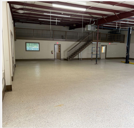
14' clear height, epoxy-coated floor
