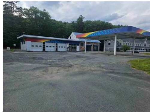
former gas station.
