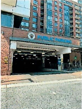
Parking garage behind the bldg.
