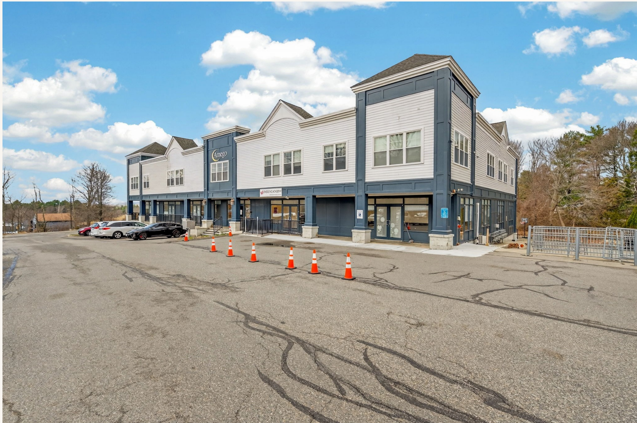
140 N. Franklin Street — Building Exterior, Holbrook MA
