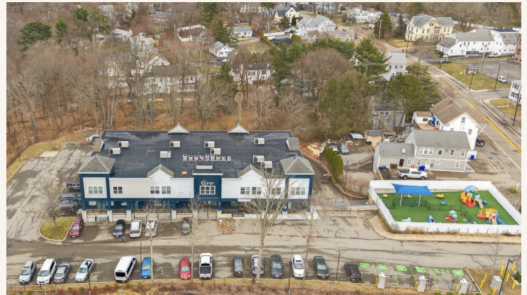
Drone Aerial — 140 N. Franklin Street, Holbrook MA
