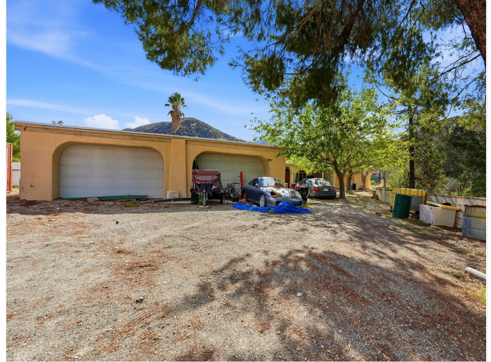
Main Home double garage
