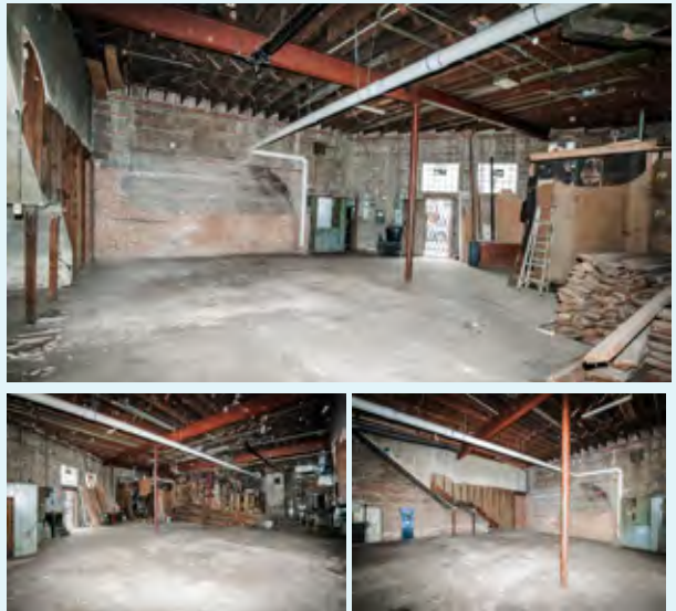
Existing Annex Conditions
