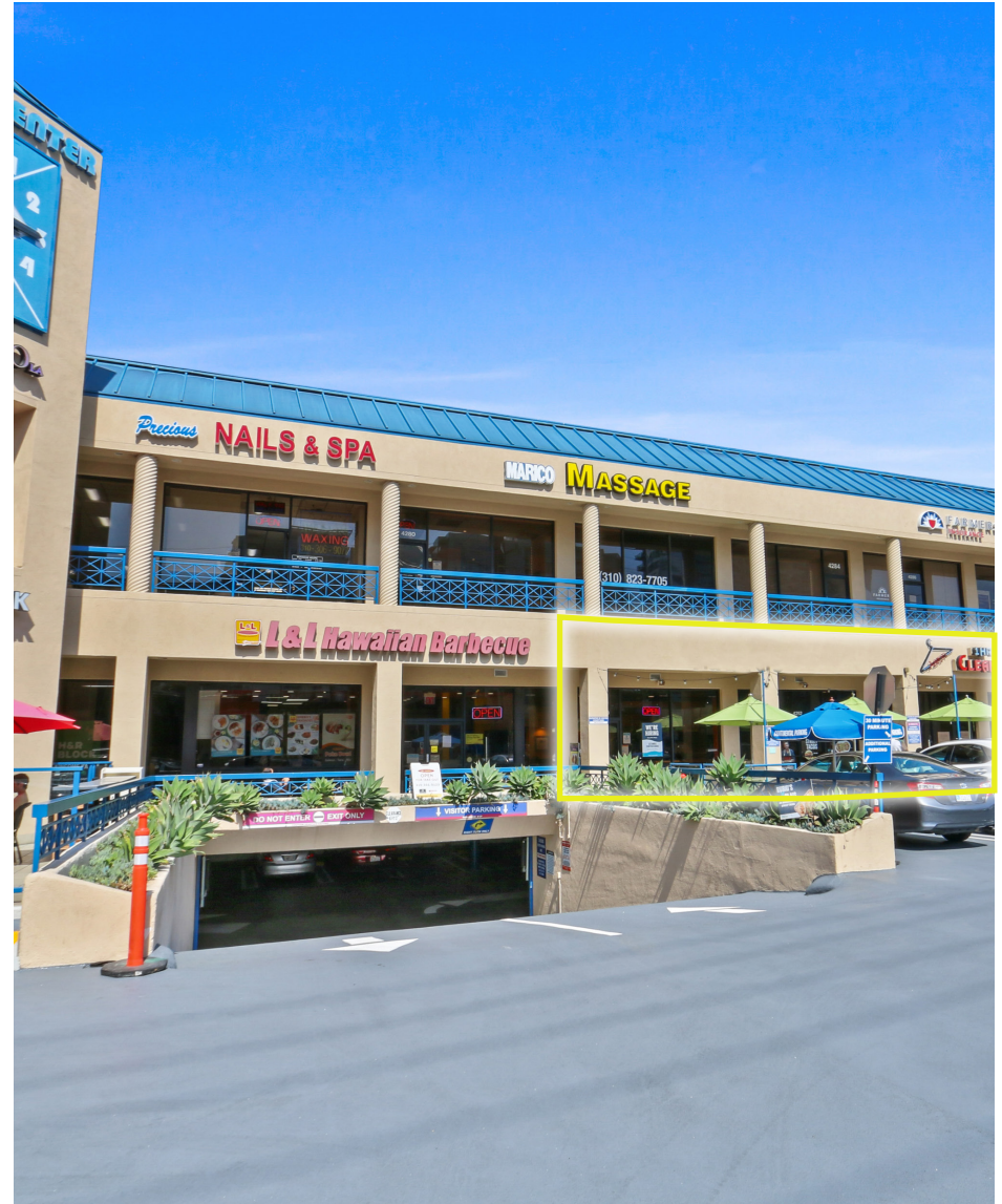
Entrance to subterranean parking
