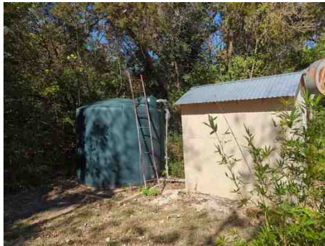
View of reservoir
