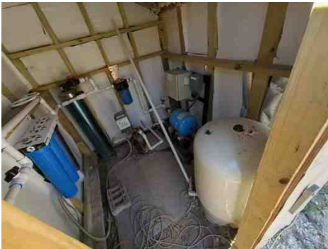
Interior of well house
