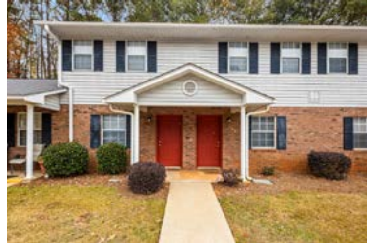
★ CHESTNUT LANE APARTMENTS 82 Berry Avenue, Newnan, GA 30263
